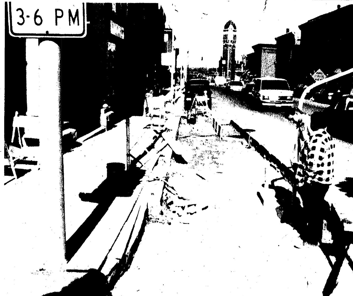
STREETSCAPE WORK began on the west side of Main St. last week, the final major area that has yet to turn up and replaced by paver blocks. Here, workers lay forms in front of the Chelsea 14th District Courthouse.
